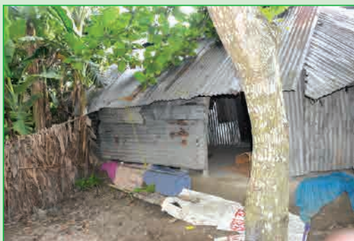
House located on khas land in Nimdi Village Patuakhali. May 2022.
